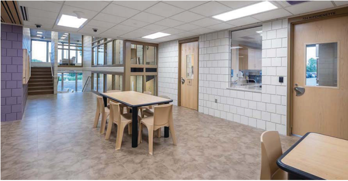
The renovated Minnesota Security Hospital in St. Peter created more than 40 patient transitional rooms and replaced an 80-bed, multi-floor area with a single-floor wing. The design added wider hallways, replaced cinderblock with clear glass, removed the carpet in favor of tiles, and placed more comfortable furniture in common areas. (Submitted Photo: Adolfsen & Peterson)
