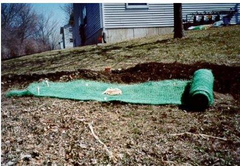
Erosion Control Blanket
